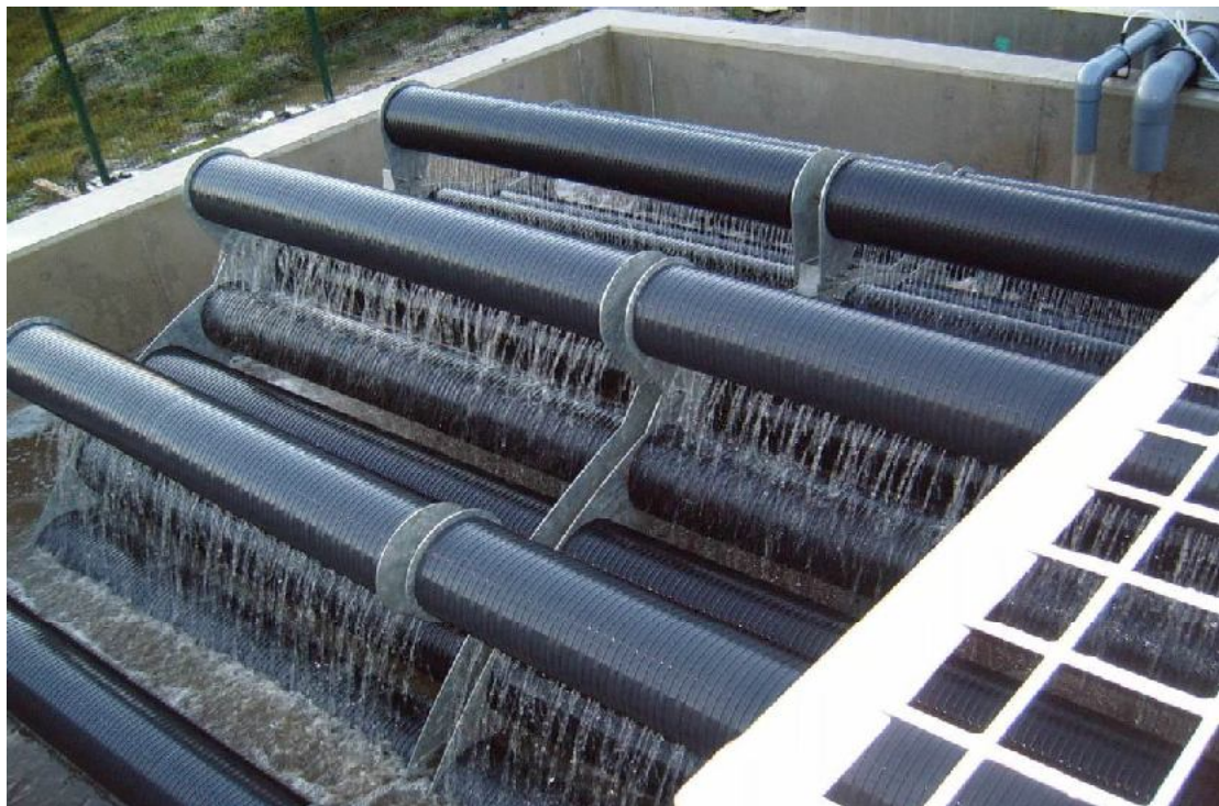
Figure 19 – Rotating Drum at Fenagh WWTP
